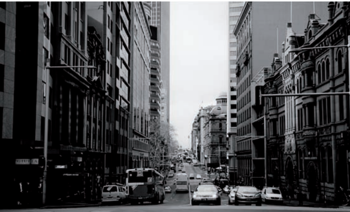
Bridge Street existing condition
